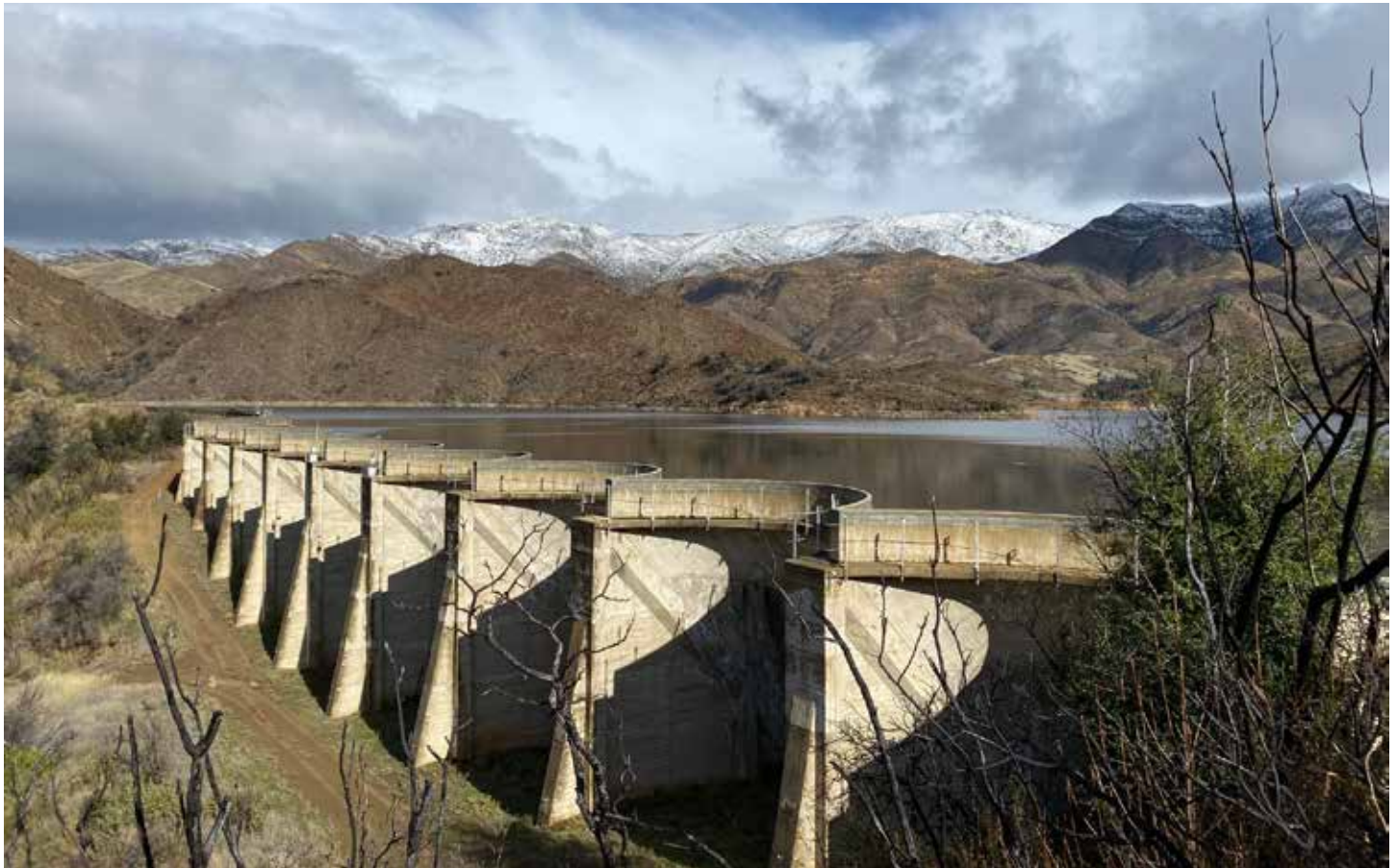
Juncal Dam at Jameson Lake, February 2020
