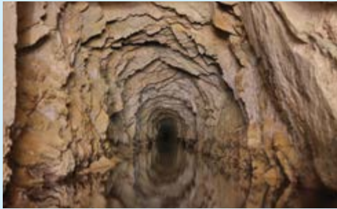
Doulton Tunnel, a horizontal well, source of groundwater and conveyance from Jameson Lake.
